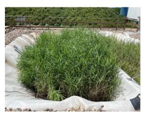
**CDSRBs** are vertical flow constructed wetlands designed to treat biological solids from upstream treatment systems such as biofilm or high rate algae pond systems. They are composed of different layers of gravel of different granulometry, and are proposed as an alternative to conventional secondary settling tanks.
