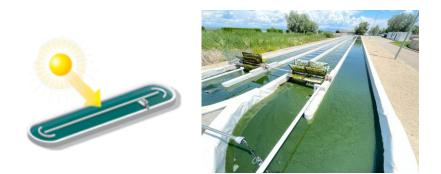
High Rate Algal Ponds (HRAP) are shallow raceway ponds that circulate wastewater via a low-power paddle wheel. In this process, a microalgae-bacteria consortium is established, where the microalgae use sunlight to carry out photosynthesis, transforming CO2 into O2, which is used by the bacteria that consume the organic matter. In addition, microalgae use nutrients (N, P) present in wastewater to grow.
